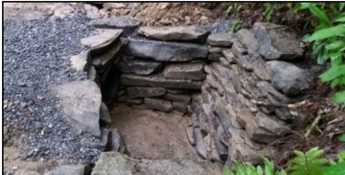
Stable headwall with bankwall
